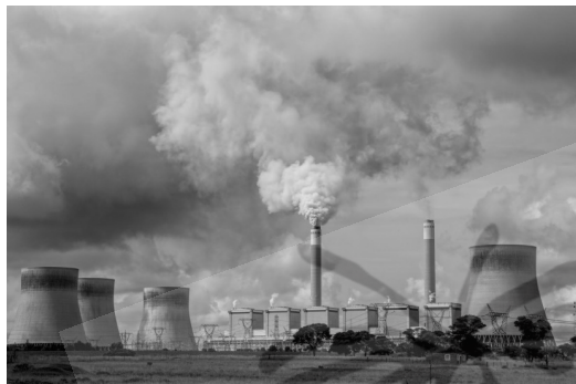
Coal-burning power station
